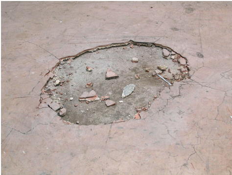
Massetto in magnesite, Suva
